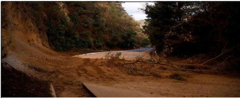
Landslides caused by earthquake in Guatemala
