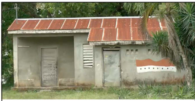
Location where chopping incident occurred
