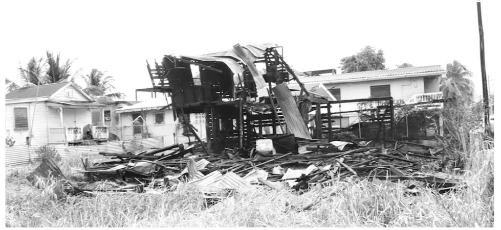
Fire on Cran Street
