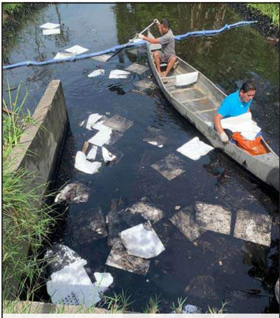
Clean-up crew working in drain affected by oil spill
